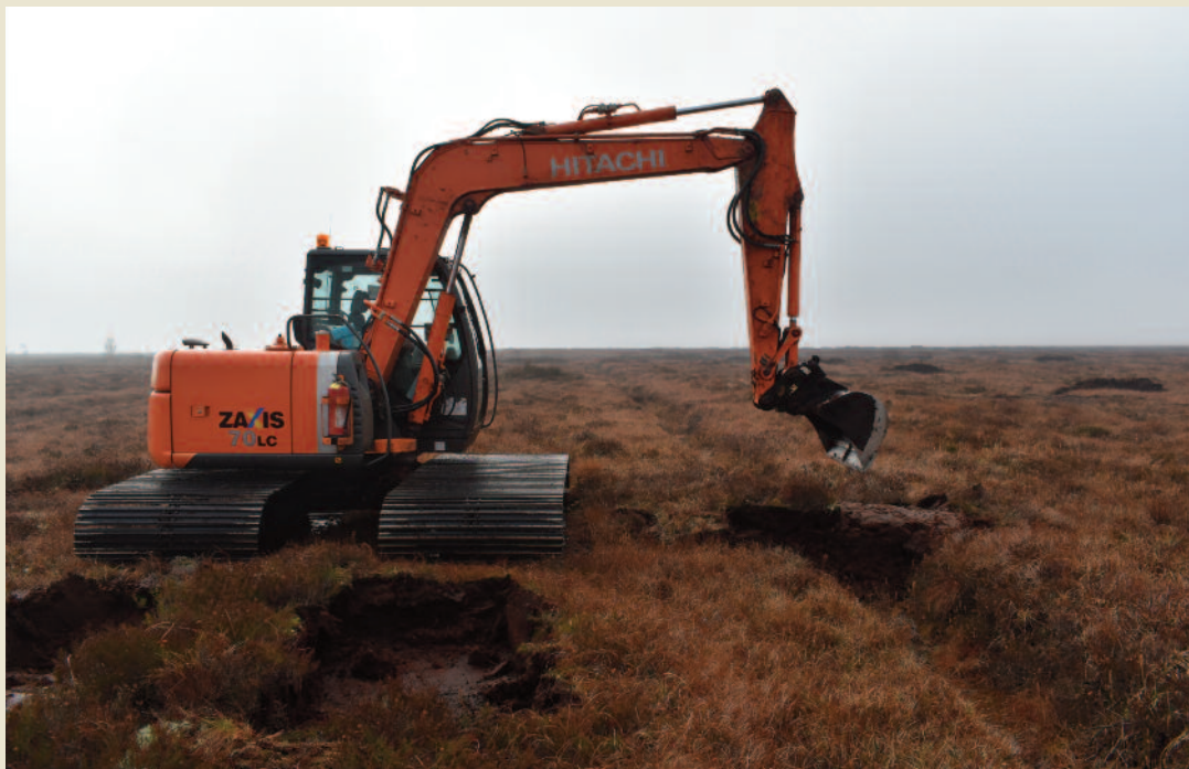
Peat dams being placed into a drain by 'The Living Bog', blocking the drain to keep water on the raised bog. For more information go to http://raisedbogs.ie/
