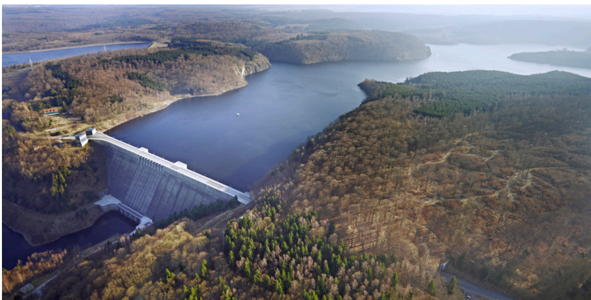
Rappbode dam, Germany. Picture: A. Künzelmann/UFZ
